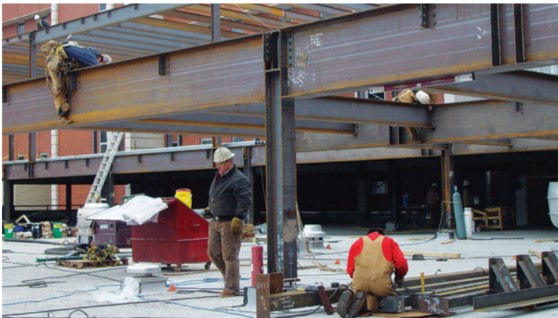
Construction teams renovated the St. Anthony Hospital in Oklahoma City. This project provided for doctors, staff, and patients advanced equipment and cutting-edge features in the hospital's facilities.
