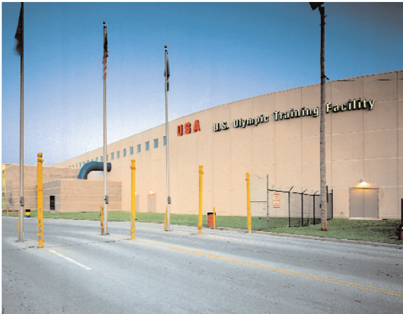
The Pettit National Ice Center keeps the air cool and dry, and the ice in peak condition, with natural gas-burning desiccant dehumidification systems.
