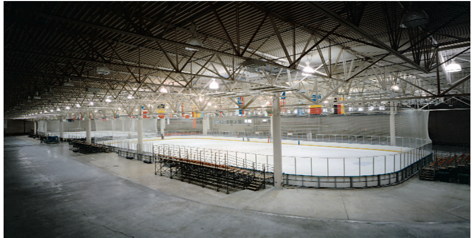
Pettit National Ice Center is one of numerous ice arenas nationwide which use cost-saving desiccant
