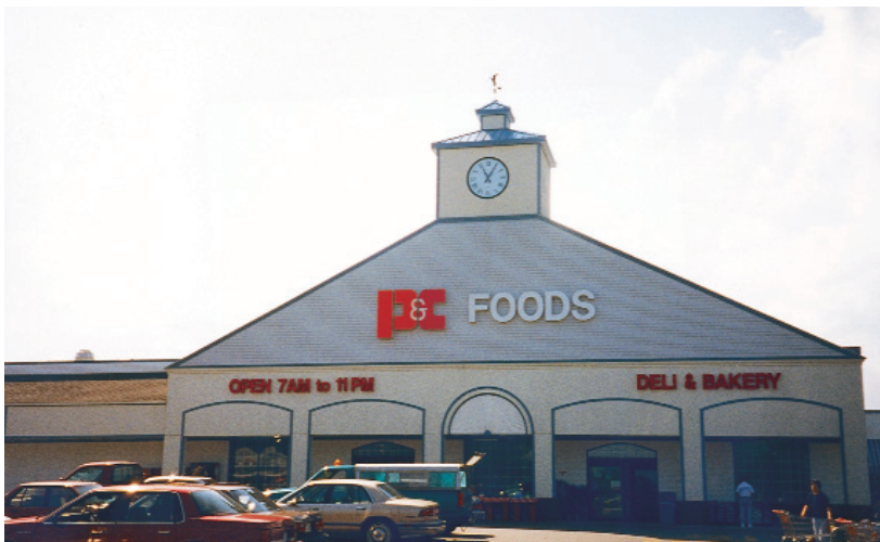
P&C Foods of Canastota, New York is one of thousands of supermarkets nationwide already realizing the significant energy savings that desiccant dehumidification systems offer.
