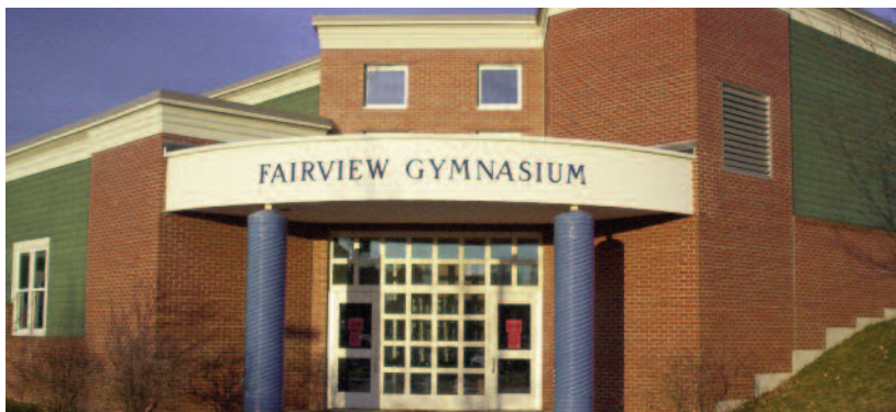
Fairview Elementary School had a serious indoor moisture problem that produced mold in classrooms and buckled an expensive gymnasium floor. Adding Munters' desiccant dehumidification equipment solved the problem.
