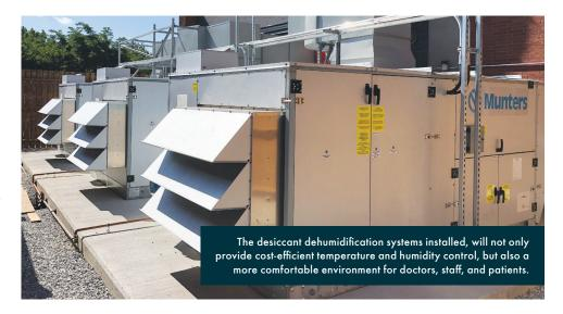
utilizes both the cooling energy from the compressor and the heat-reclaim to regenerate the desiccant rotor (exceeding the criteria of ASHRAE 90.1). Building operators bring the new dehumidification systems on-line whenever the outdoor ambient conditions rise above 5°C/41°F – ensuring the critical spaces will always maintain the required low dew points.
